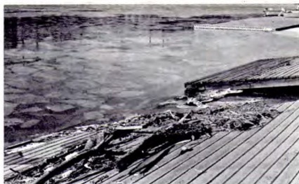
Ravages of winter -- the UBC ramps lie alone after ice and high water carried our float over the dam. Plans for the new float construction include filling in the gap between the old ramps and replacing the floatation at the lower end. The use of pressure-treated lumber is expected to vastly increase the life of the new float. The club is indebted to David Rawle for his efforts in obtaining and expediting delivery of the wood.
