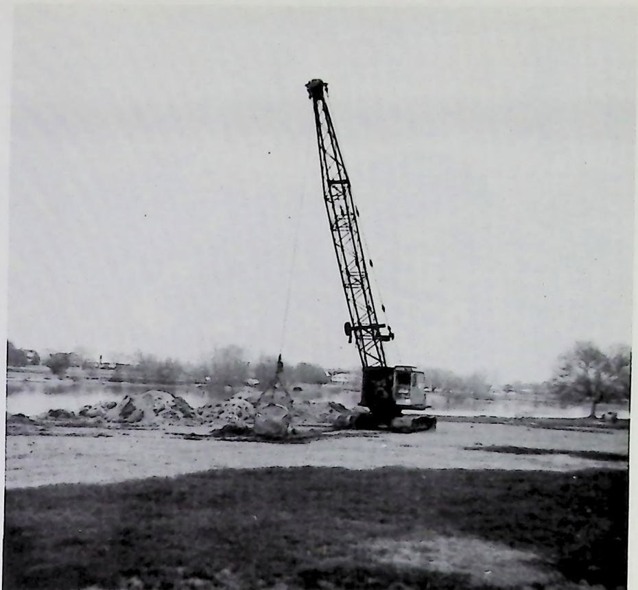
1½ yard drag line in action cutting along south shore of Camden's Cooper River. Above picture shows one of the four dredges preparing the course for requirements of the International Rowing Foundation (FISA).
