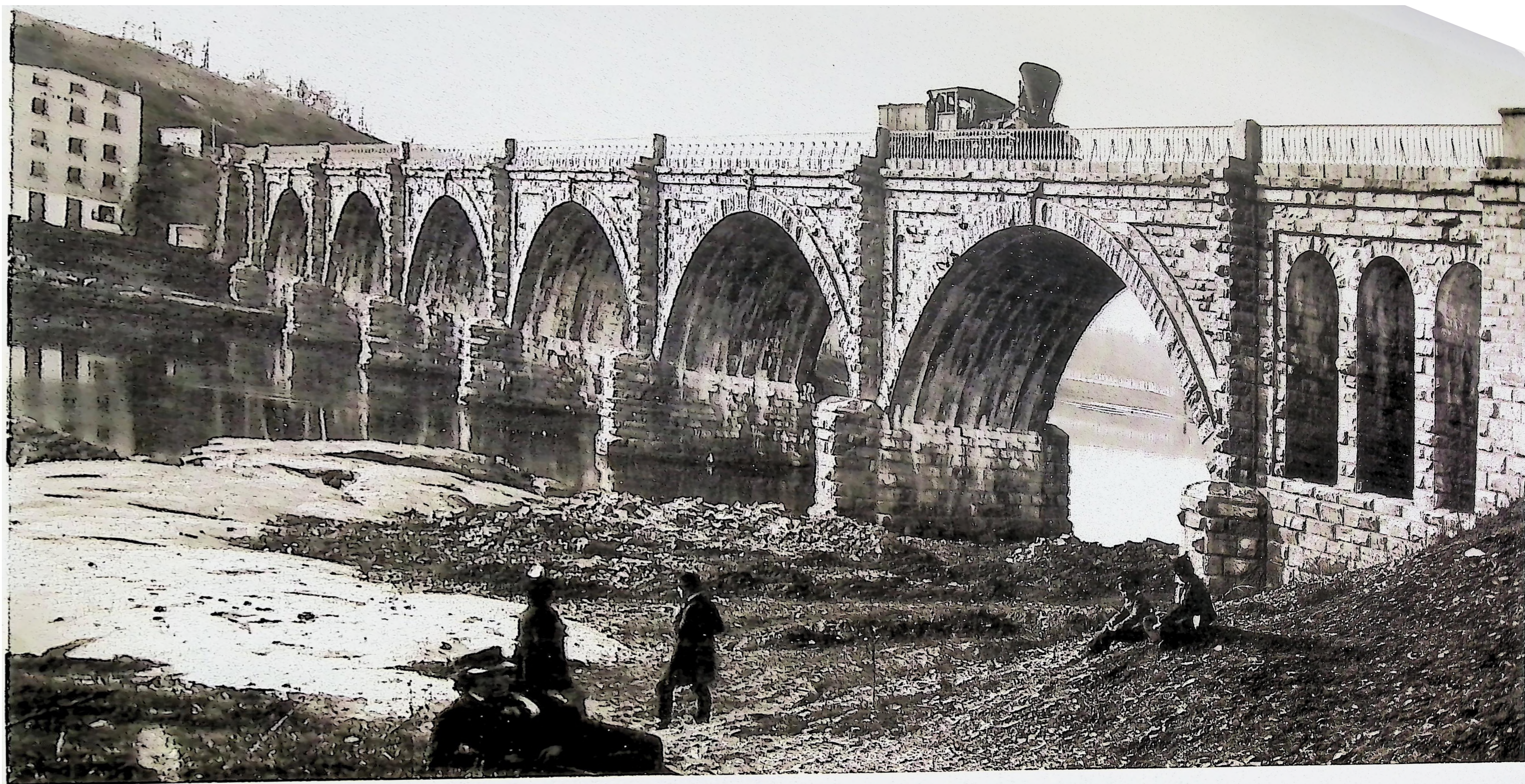
COLUMBIA AVE BRIDGE - 1870?
